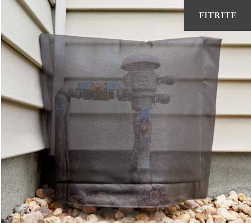
BACKFLOW ASSEMBLY WITH COVER
